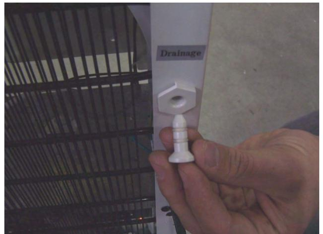
9.2 Drain any remaining water in the system by depressing the faucets.
